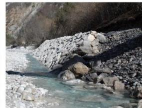
ESEMPI DI RIFACIMENTO/RIPRISTINO ARGINATURA SPONDALE CON SOGLIERA "A MASSI SCIOLTI" UTILIZZANDO I MASSI E TROVANTI IN LOCO PRESENTI IN ALVEO
